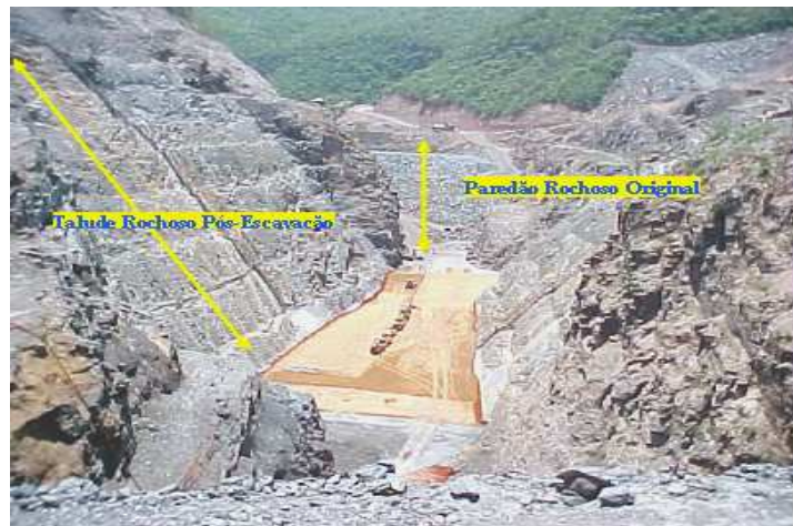
Figure 2. Core dam – Excavation for geometric improvements.
