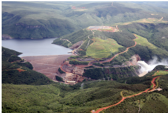
Figure 3. Panoramic of the completed dam
